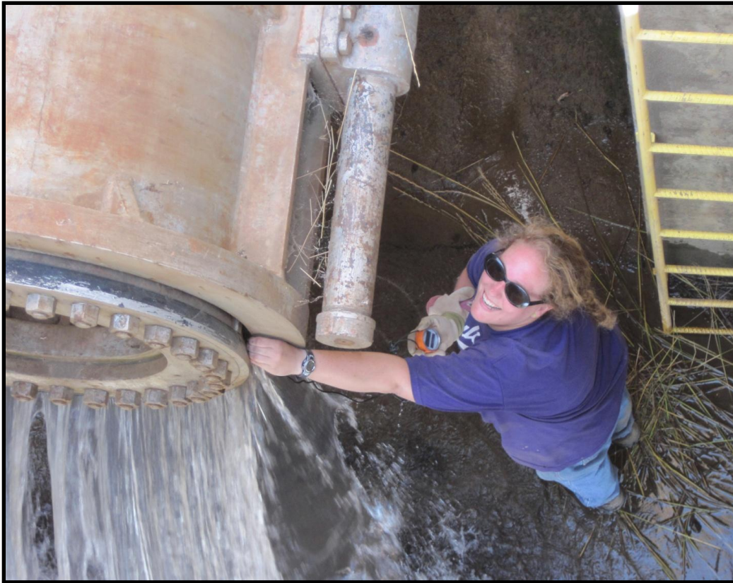
Bridget Bergiel checking the water temperature at the Howell-Bunger valve at the Mill Creek, Bennington Lake Embankment Dam.
